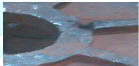
Figure 2: shows the shrinkage defect obtained due to improper riser design.
